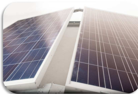
Optimized air gap at the east/west system
